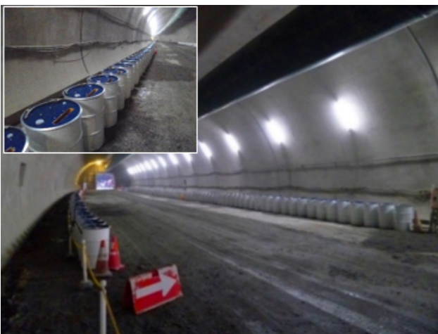
Actual installation of the Drum Silencer System
